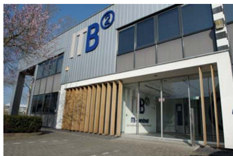
ITB2 Datacenter Deventer
